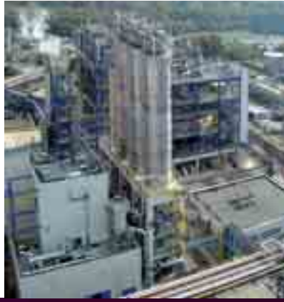
250,000 t/year HDPE plant SABIC Polyolefine GmbH, Gelsenkirchen
