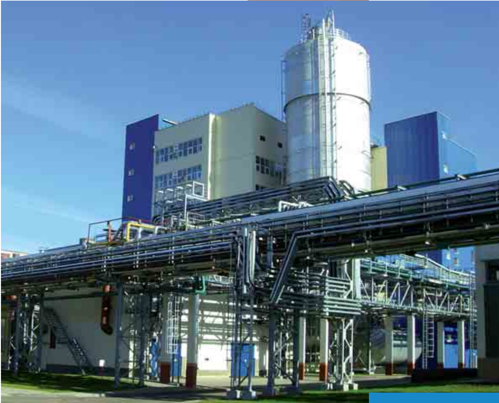
2-reactor plant for textile grade PET in Belarus which can use both PTA and DMT as a raw material
