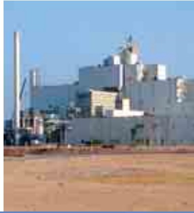
2-reactor Melt-To-Resin MTR® plant in Oman for APET sheet production
