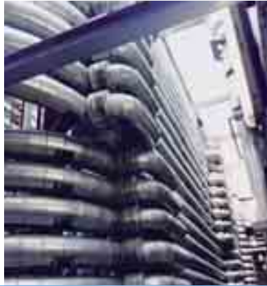
High-pressure pipe reactor for LDPE
