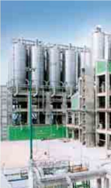
300,000 t/year HDPE plant Jam Petrochemical Co., Bandar Assaluyeh, Iran
