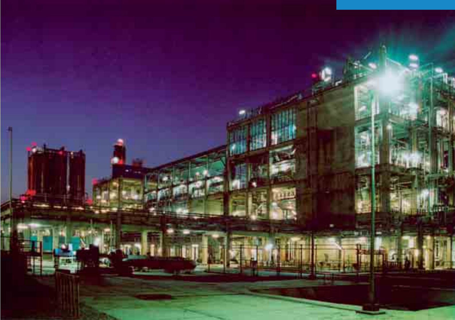
300,000 t/year HDPE plant Marun Petrochemical Co., Bandar Imam, Iran
