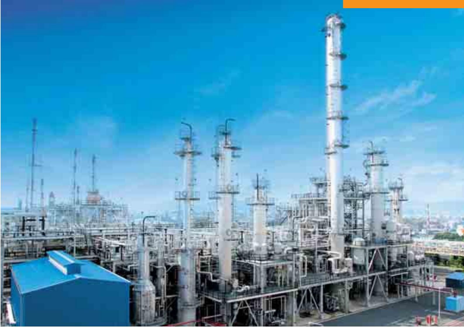
World's first HPPO plant successfully in commercial operation since 2008
