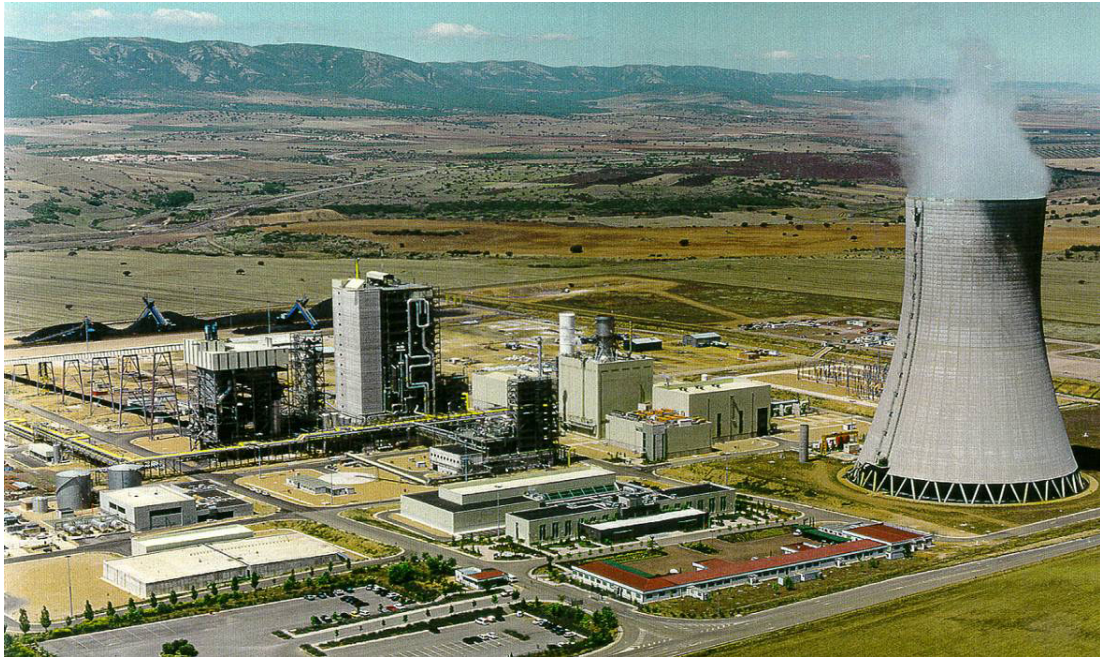
Figure 1: IGCC plant in Puertollano/Spain
